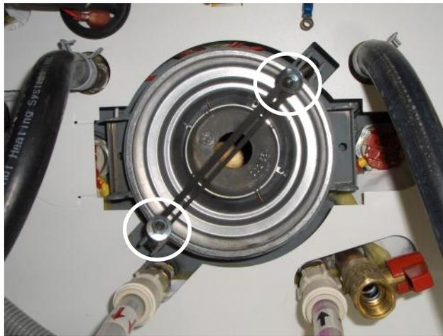
1. The Diesel-Burner is secured to the Aqua-Hot with two eye-bolt nuts that can be swung into place, after the diesel burner has been properly aligned and set in place.
