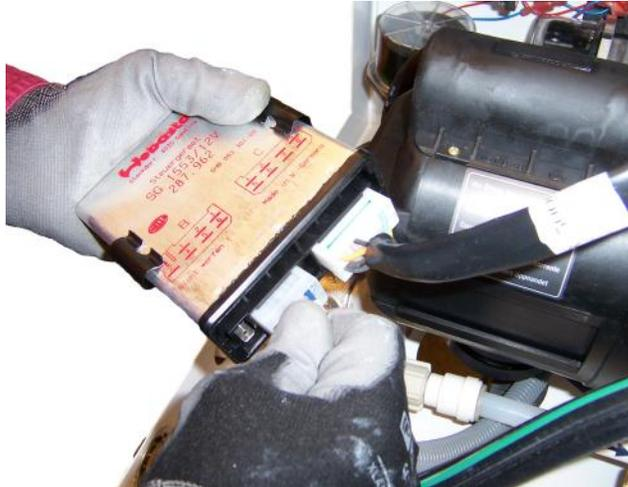
1. Locate the Diesel-Burner's Controller and disconnect both plugs. Failure to do so may result in the Diesel burner igniting.
