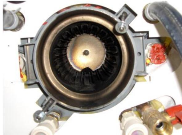
1. Remove the combustion chamber by pulling it straight out, approximately 16 inches.
