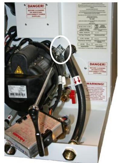
2. The eye-bolt nuts can then be tightened by using a 10mm socket wrench with a 10 inch long extension. Use extreme caution when tightening down the eye-bolt nuts, over tightening of the eye-bolt nuts can cause the aluminum blower casing to crack. (Torque Specifications = Approximately 20-40 in. lbs.)
