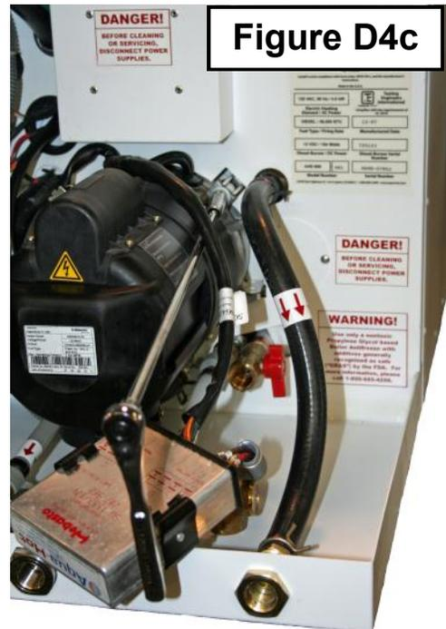
3. The Diesel-Burner is secured to the Aqua-Hot with two 10mm nuts that can be loosened, and swung out of the way by using a 10mm socket wrench with a 10 inch long extension.
