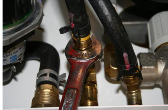
1. Align the fuel lines on the diesel burner with the fittings on the Aqua-Hot, and using a 11/16 inch wrench, tighten down both the supply and return fuel fittings.
